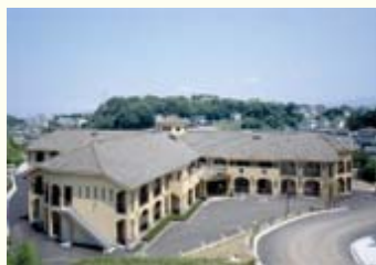
Fireproof Structure Example – Meiji Sei-Ryu-En Oita Prefecture, Kyushu Floor Area:
