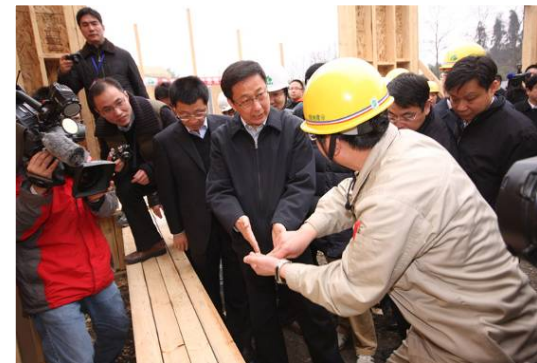
Top: The main building of the Xiang'e school complex. Bottom: Mayor Han of Shanghai is followed by news cameras as he visits the Xiang'e project site. Both photos - February 9, 2009.
