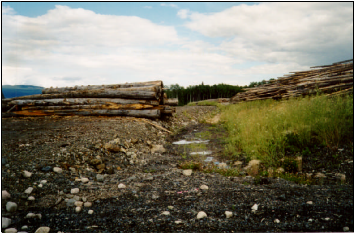
PHOTO4: Portion of log yard at Fraser Lakes showing typical "terrace" and drainageditch.
